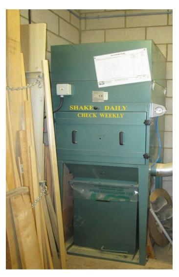
Once the installation was complete and to prove that the new LEV effectively controls the dust levels, emitted by the additional machinery, to as far below the WEL (Workplace Exposure Limit) as is reasonably practicable, P&J's LEV engineer attended site to commission the new set up.
